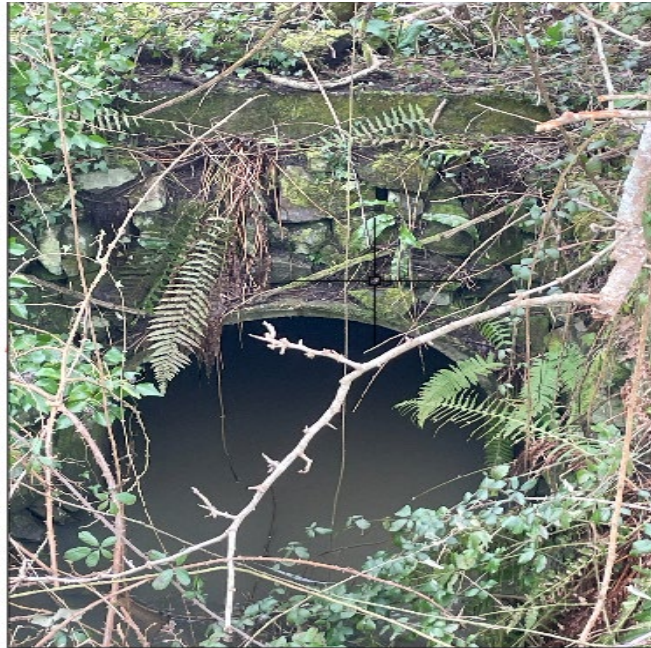
Figure 2.2 Culvert beneath Tarka Trail
