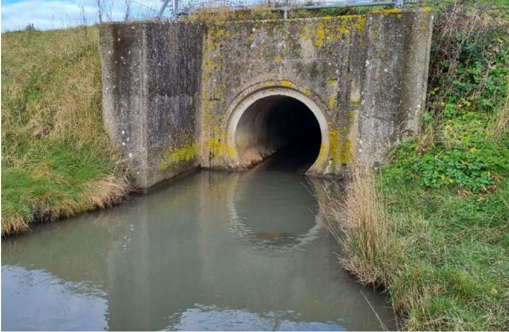
Figure 2.4 Outfall Culvert into Taw Estuary
