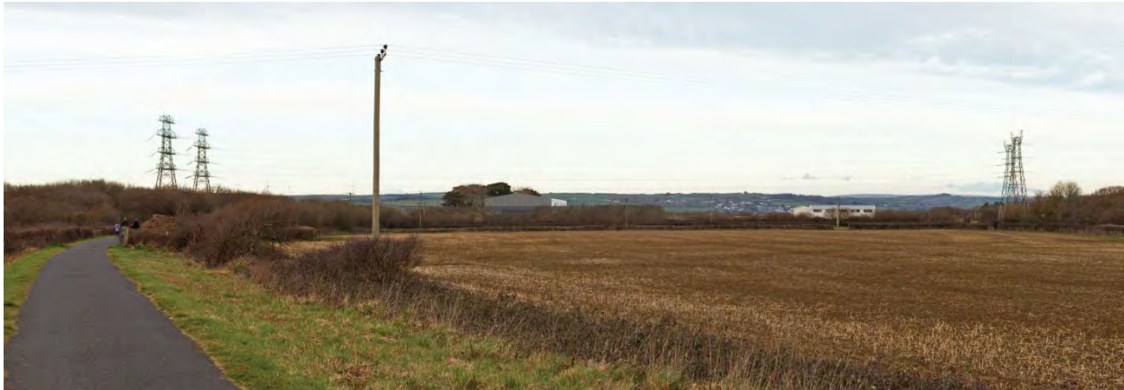
Photo 5: View of the White Cross Onshore Substation from the north-west, illustrating the “stepped” massing of the Substation building and Control Room building. (Submitted Elevation Viewpoint 1, 15 years vegetation growth).
