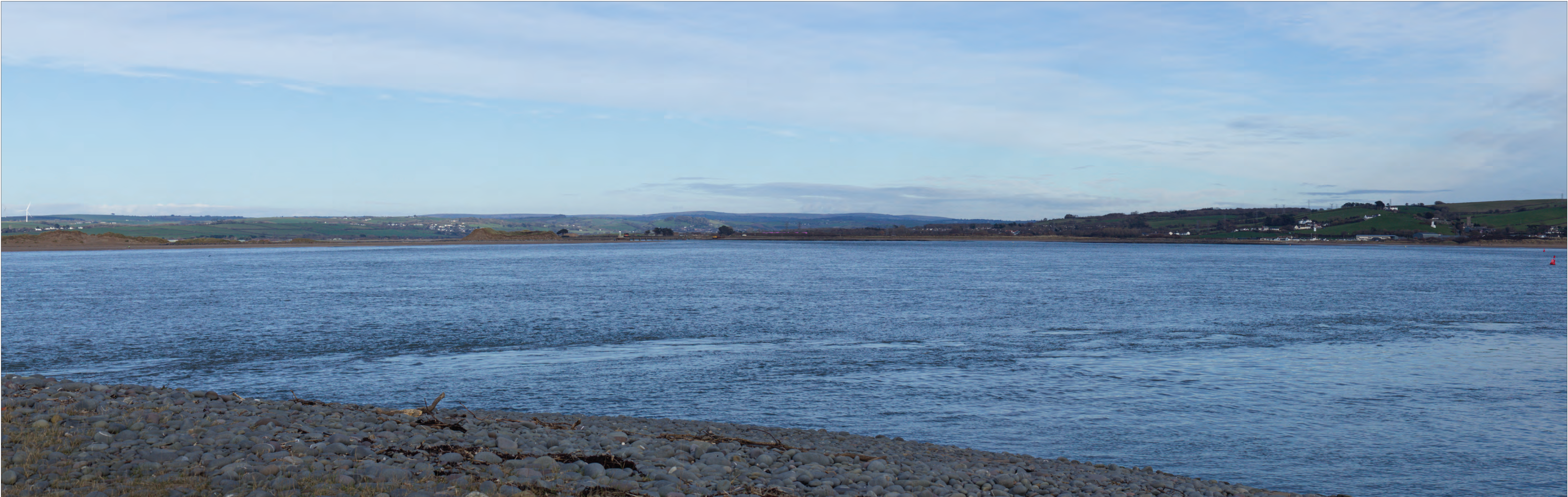
OS reference: 245329E 131449N Horizontal field of view: 53.5° (planar projection) Camera: Canon EOS 6D Enlargement Factor: 150% @A1 Figure 20:21c / PC2978-OPN-ZZ-XX-DR-Z-0645c - Proposed Onshore Substation WCS Maximum Parameter with Mitigation Planting (0 Years Growth) Eye level: 5.54 m AOD Principal distance: 812.5 mm Lens: Canon EF 50mm f/1.4 Viewpoint 8: Greysands Hill (Northam Burrows Country Park), on SWCP Direction of view: 76° Paper size: 841 x 297 mm (half A1) Camera height: 1.5 m Date and time: 07/03/2023, 16:23:14 White Cross Offshore Wind Distance to site: 2.86 km Correct printed image size: 820 x 260 mm
