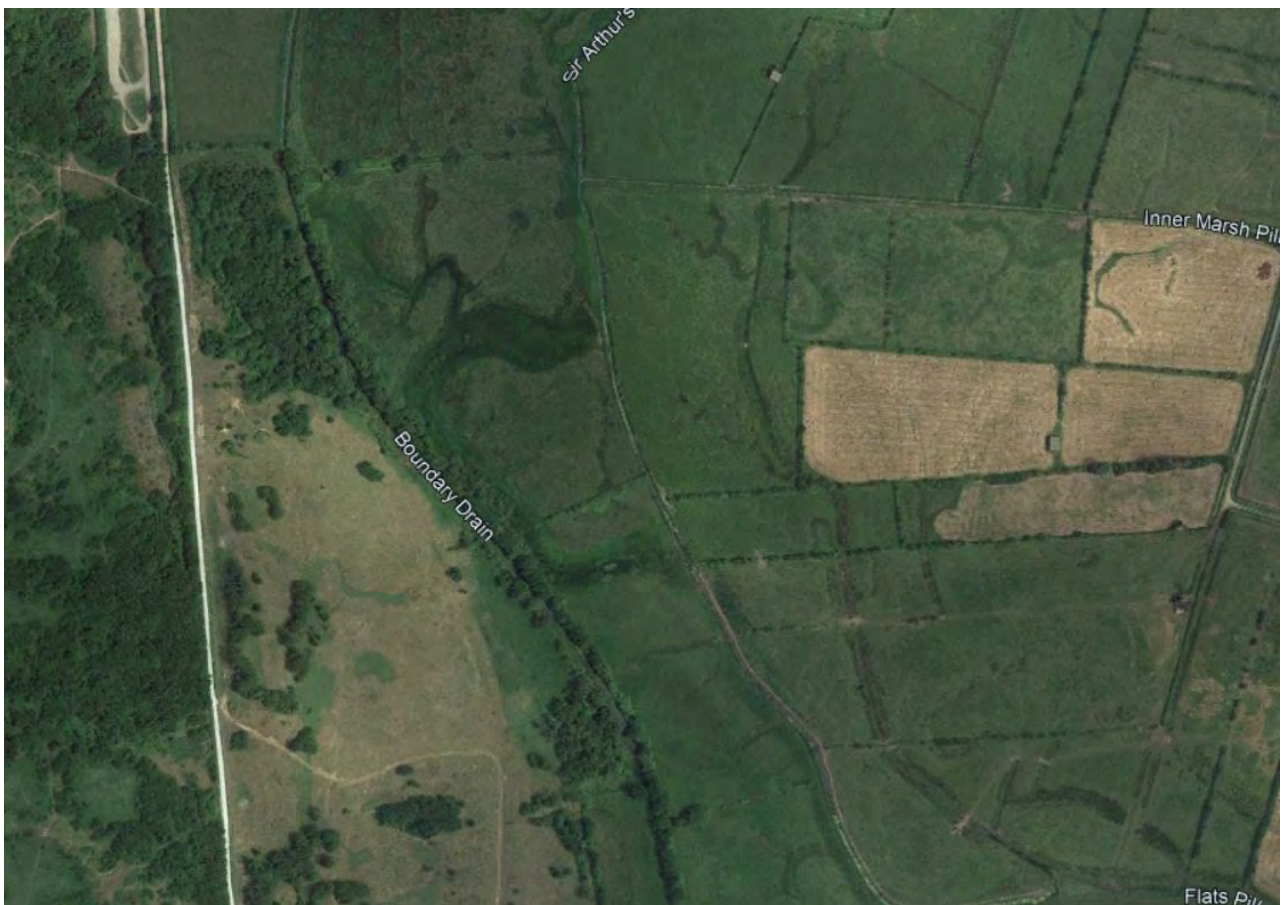
Plate 9: Branton Marsh in 2022, from Google Earth, modern appearance following drainage of the marsh
