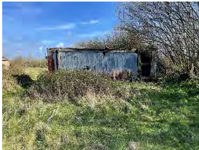
Figure 2.6. The north-western elevation of the Lean-to at South Barrow Farm
