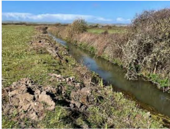
Pond 54 – Boundary Ditch South
