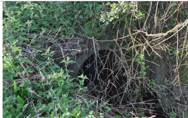
Plate 3.38 Small culvert on the main drainage channel.
