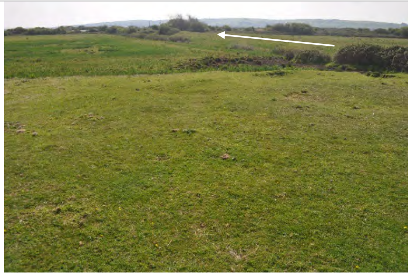
Plate 3.18 Floodplain embankment (indicated by white arrow).
