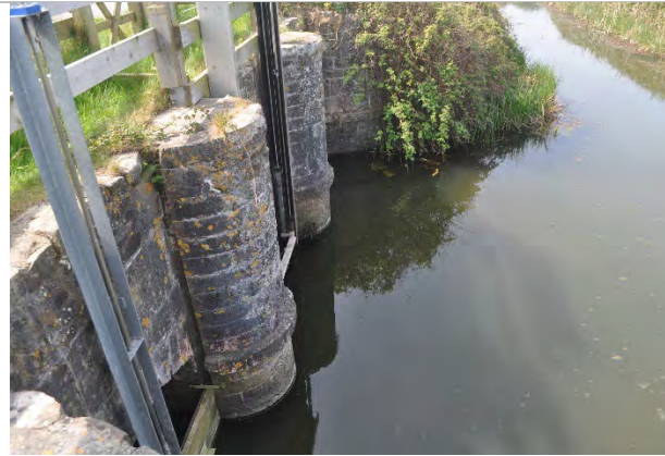
Plate 3.11 Boundary Drain on upstream side of the Great Sluice.
