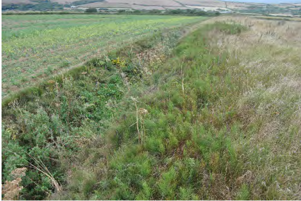
Plate 3.27 Typical incised drainage channel crossing arable fields near Saunton Golf Course.
