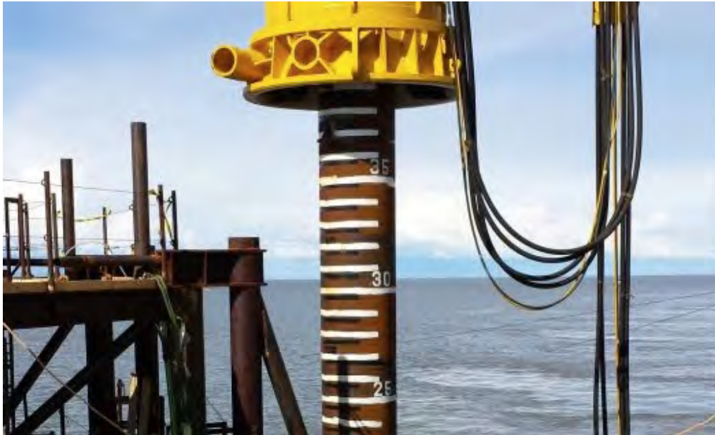
Plate 3.9 Driven Pile Example (Pile.com, 2022)
