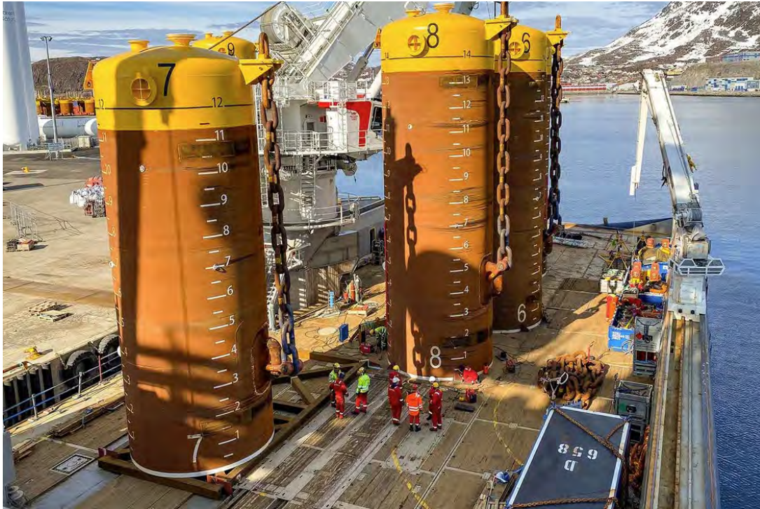
Plate 3.8 Suction Anchor Example (Source: Offshore-Engineer, 2020)
