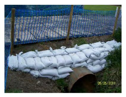
Plate 5.6 Typical culvert crossing for minor watercourse
