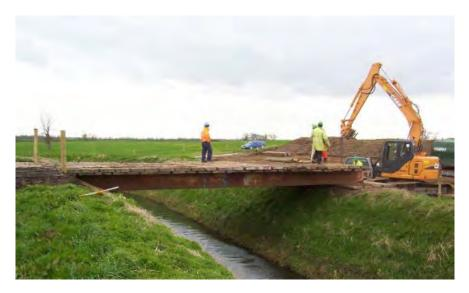
Plate 5.7 Typical beam bridge crossing for larger watercourse
