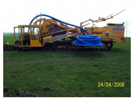
Plate 5.9 Pre-construction drainage being installed using drainage trenching machine
