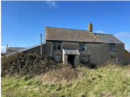
Figure 2.2. The south-eastern elevation of South Barrow Farmhouse
