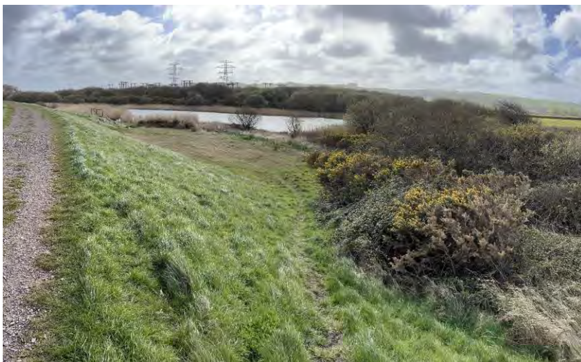
Photograph 1-2. The Yelland coastal embankment including coastal grassland & scrub
