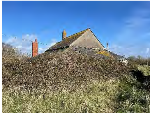
Figure 2.3. The south and north-western elevations of South Barrow Farmhouse
