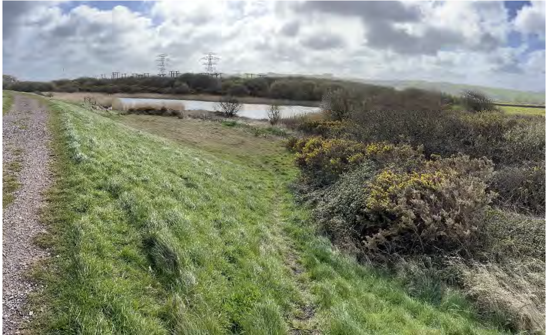
Photograph 3-33. The Yelland coastal embankment including coastal grassland & scrub
