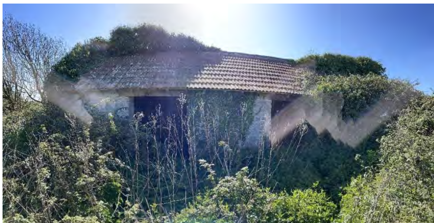
Figure 2.1. The southern elevation of Braunton Barn
