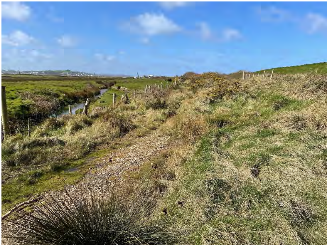
Photograph 3.34. The Yelland coastal embankment including coastal grassland & scrub
