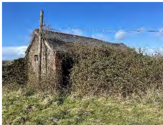
Figure 2.5. The south-western and south-eastern elevations of South Barrow Barn
