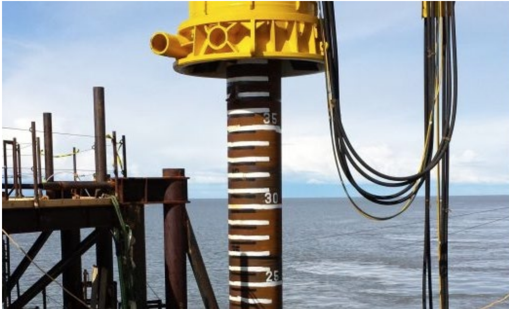
Plate 3.9 Driven Pile Example (Pile.com, 2022)
