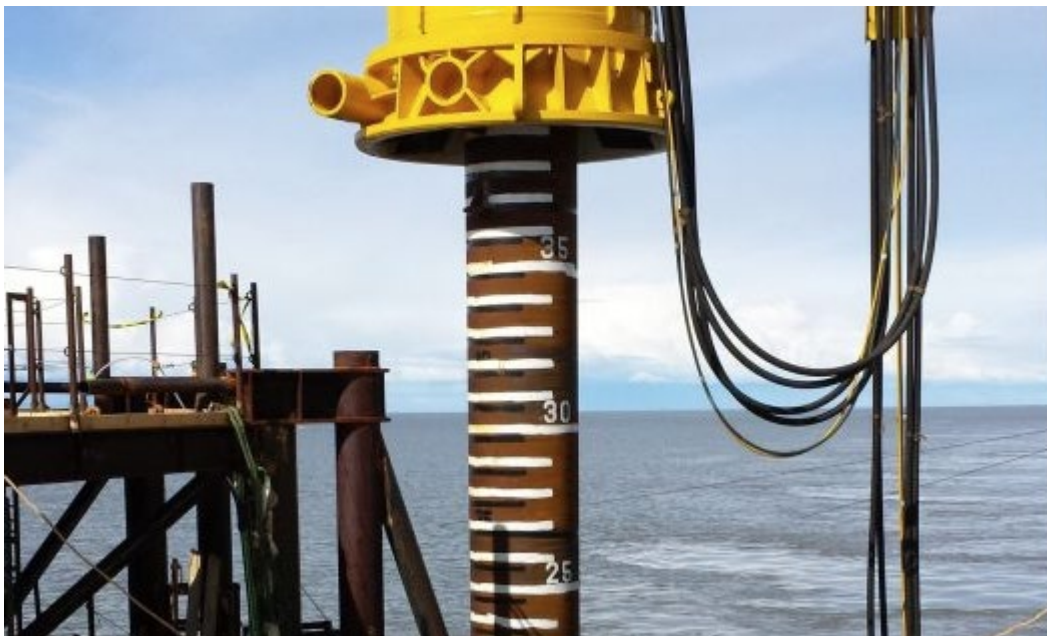
Plate 5.9 Driven Pile Example (Pile.com, 2022)
