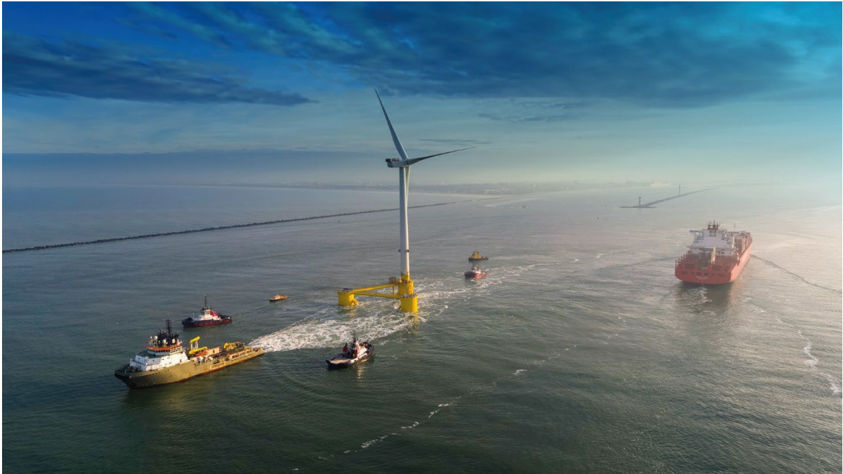
Plate 5.14 Tug vessel towing the Kincardine's integrated WTG and semi-submersible substructure unit out to Windfarm Site.
